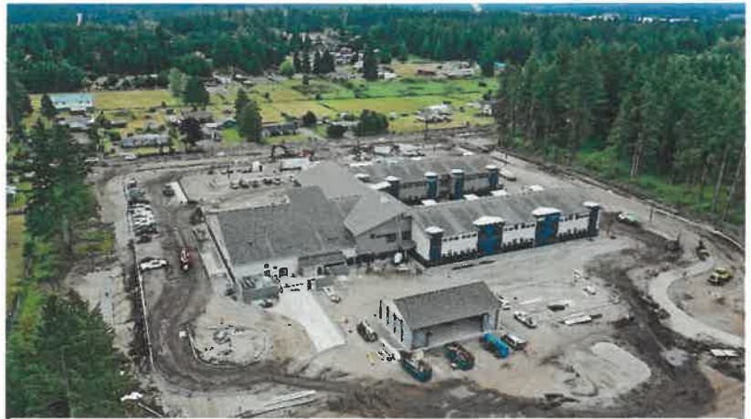
Katherine G. Johnson Elementary under construction
