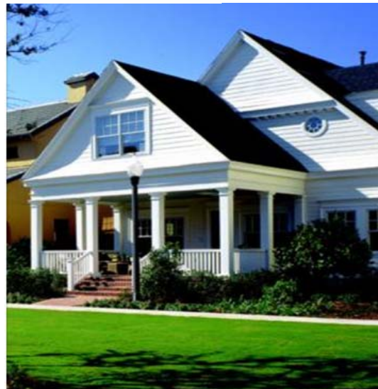
Figure 2-6: Desirable: Front Yard without garage or parking apron. Alleys are desirable to eliminate the impact of the garage door & driveway on the streetscape and eliminate access conflict to the street
