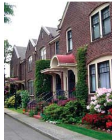
Figure 3D-21A: Visible building entry
