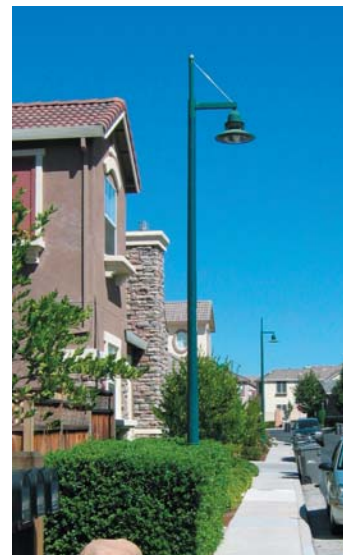
Figure 3D-26: Encouraged: Pedestrian-scaled decorative light fixtures add to the intimacy and character of a neighborhood.
