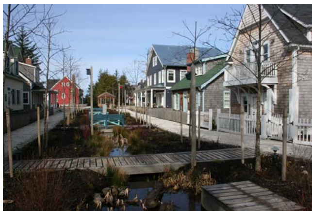
Figure 3A-3C: Single-family homes in Seabrook oriented to linear park stormwater feature
