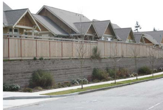
Figure 3A-2B Undesirable Design: Houses separated from the street by high solid walls
