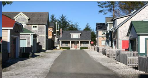
Figure 3A-18B Garages in Seabrook, some with second floor ADUs, located in a rear alley
