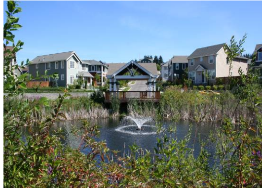
Figure 3A-6: Storm pond amenity located at The Commons
