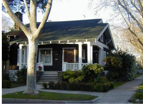
Figure 3B-12A: Entry porch highlights primary entry to the house and is oriented toward the street
