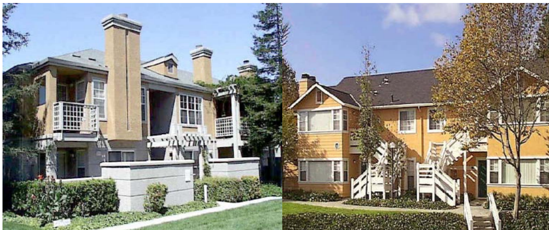
Figure 3D-18A: Individual residences are articulated through the use of variation in the massing, recessed balconies, wall breaks and varying roof forms.
