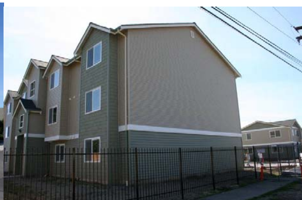
Figure 3D-22B: Undesirable: Building presents a blank wall lacking articulation, modulation, or window and door openings, to the street.
