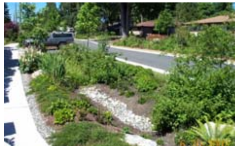
Figure 3D-7 Vegetated bioswale
