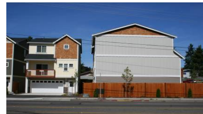
Figure 3D-2: Undesirable: Buildings with blank walls or with lack of articulation facing the street
