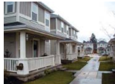
Figure 3B-13: Use of porches can help transition from the public to the private realm and create a space for residents to congregate.
